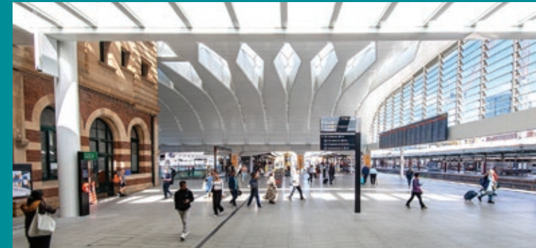
Central Station's upgraded Northern Concourse with transformed pedestrian thoroughfares and feature roof. Image: Sydney Metro.
